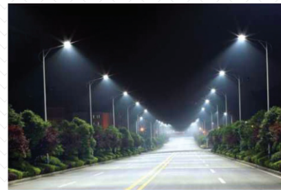
LED Street Lights
